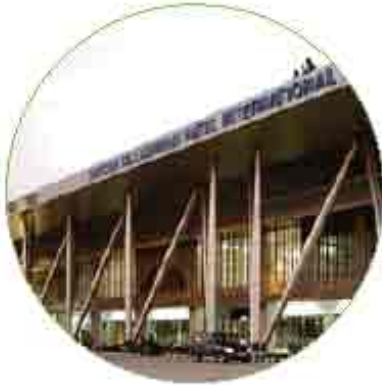
Sardar Vallabhbhai Patel International Airport Ahmedabad, Gujarat
